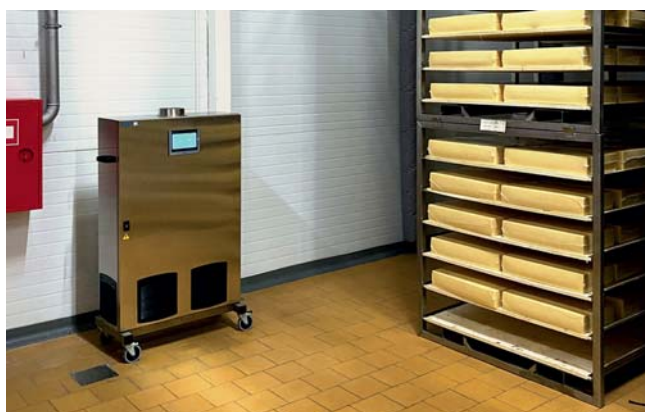
FIGURE 3. «AEROLIT-1000» recirculator in the cheese maturation chamber
